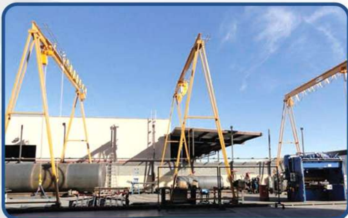
Three track mounted PS Series Gantry Cranes mounted over rail cars for easy maintenance and repair. The track mount ensures smooth travel over a fixed route for increased productivity and ease of use.
