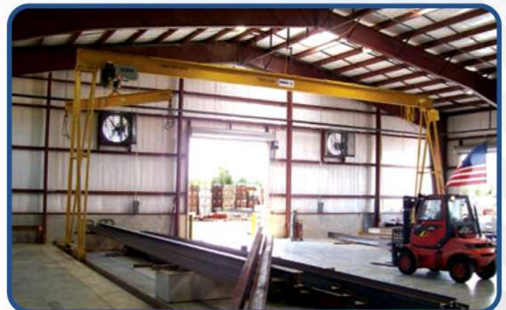
A 7.5-ton Motorized Verkrönn PS Gantry Crane used to move truckloads of long steel beams at a building material supply center.
